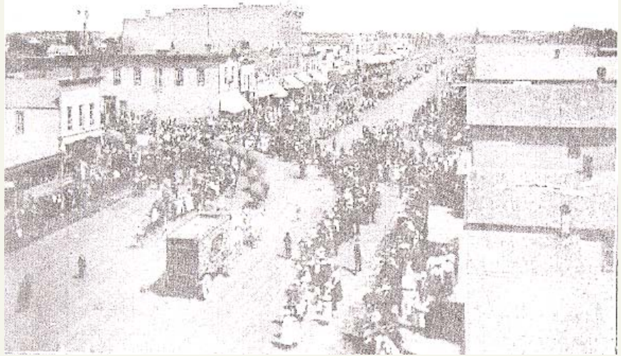
The 1892 circus parade turns west on the corner of South Egan and S.W. 1 st to the show grounds several blocks west.
